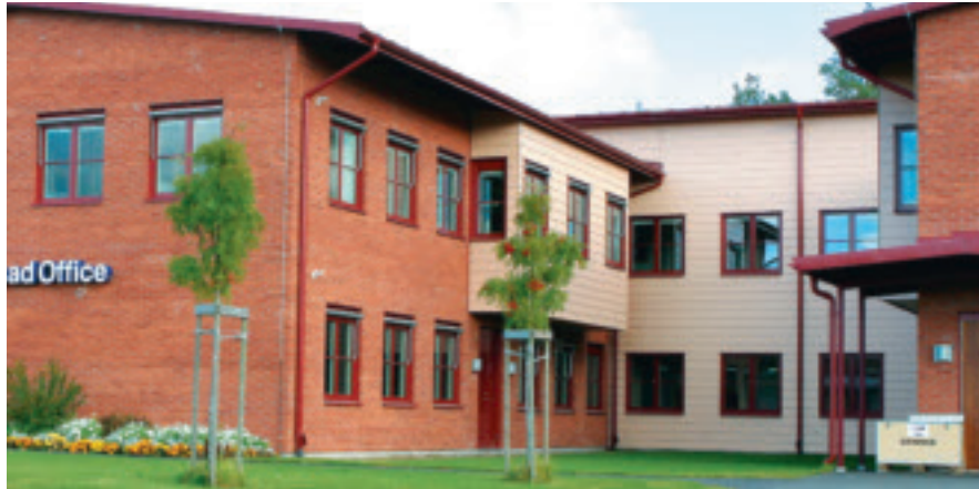
Office building with Formica Exterior installed as weatherboarding, Oskarshamn, Sweden.
