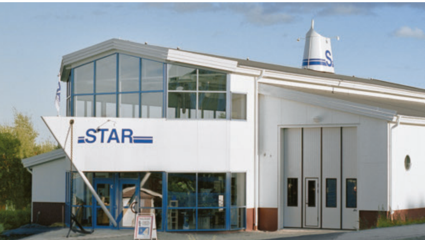
Office building in Västervik, Sweden
